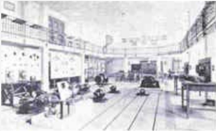
(1935) ELECTRIC MACHINES LABORATORY
